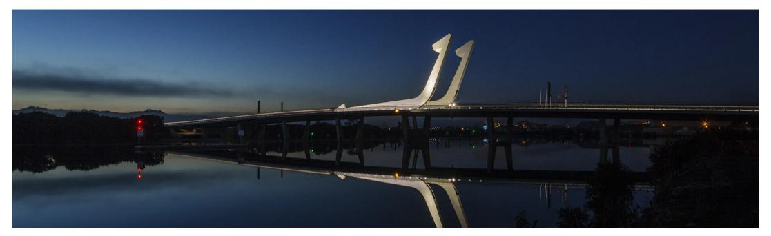
The challenge was to highlight the "J" shaped fish hook primary structure to create a night-time iconic image for the new crossing, while providing the necessary highway authority requirements for the various bridge users and considering the local dark sky environment as a natural resource.
